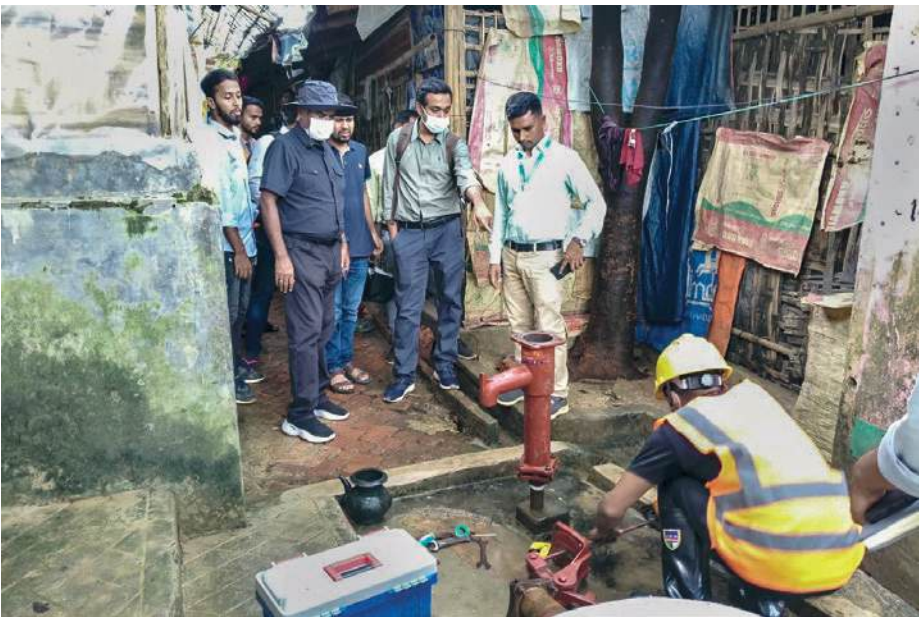
Mr. Clarence Sutharshan Sukunadas, Country Director of Tearfund Bangladesh, monitors tube well repair works at Camp 15 on August 8, 2025.
